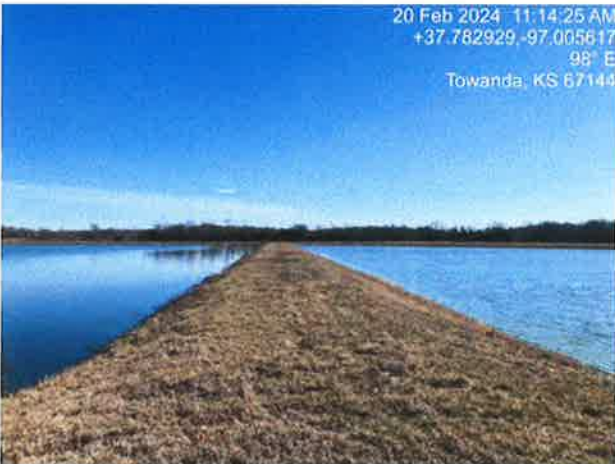
Photo Taken: 2/20/2024 11:14:25 AM Looking at Cell 2 (left) and Cell 3 (right).
